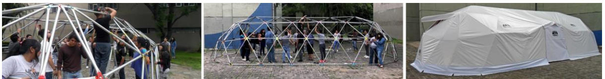
Fig. 6: Assembly of the temporary structure with rectangular base.
