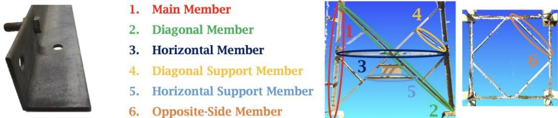
Fig. 1: Members of steel tower: (a) Angle steel and (b) Classification of steel members.
